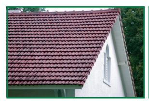
Note how the material and form of this historic clay tile roof is an integral element of the design and character of this house. Both the roof's form and its material are significant features.
