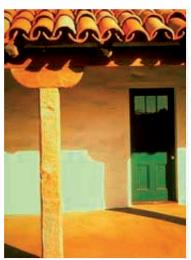
Tapered barrel clay roof tiles were custom made for the restoration of the 1820s Indian barracks at Mission Santa Cruz in California.
