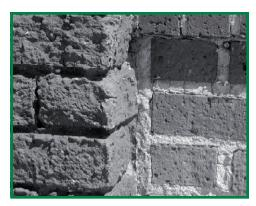
Abrasive cleaning can damage the exterior surface appearance of historic masonry.
