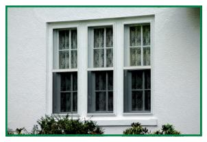
Note how the dividing rails of these storm windows meet the dividing rails of the historic window. The minimal framing is finished to match the adjacent window trim. The result is a storm window that has minimal visual impact on the historic window.
